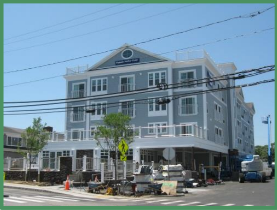
New Hyannis Harbor Hotel Under Construction
