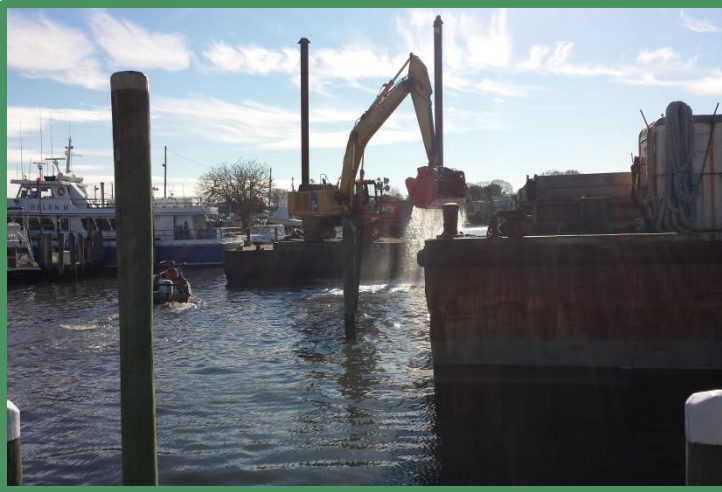
Gateway Marina Dredging Project
